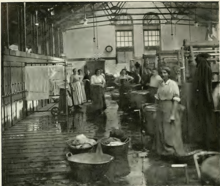
INTERIOR—SIMON SQUARE WASH-HOUSES, EDINBURGH
